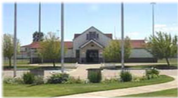
FCI Sheridan in Oregon is a medium security facility for male offenders.
